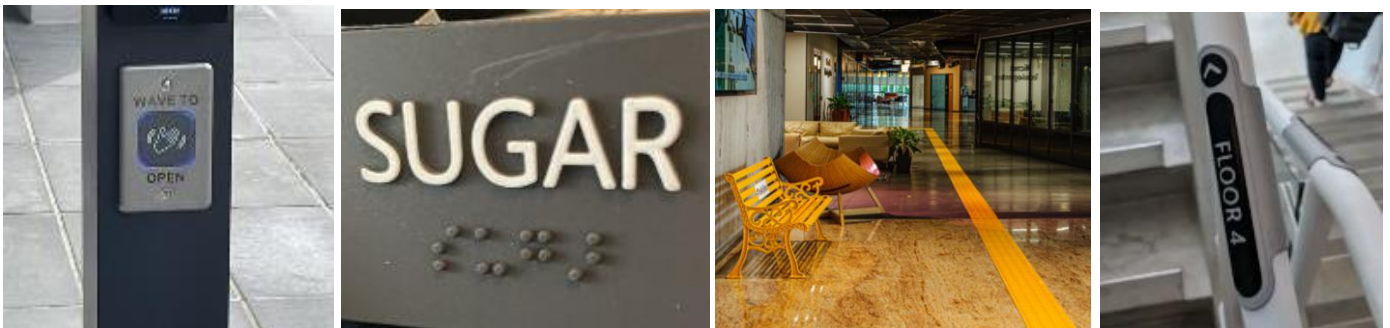
Left to right: Wave to open door entry; high contrast, braille signage in kitchenettes; high contrast, tactile floor and railing markers
