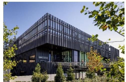
The Thermal Energy Center on Microsoft's Redmond campus.
